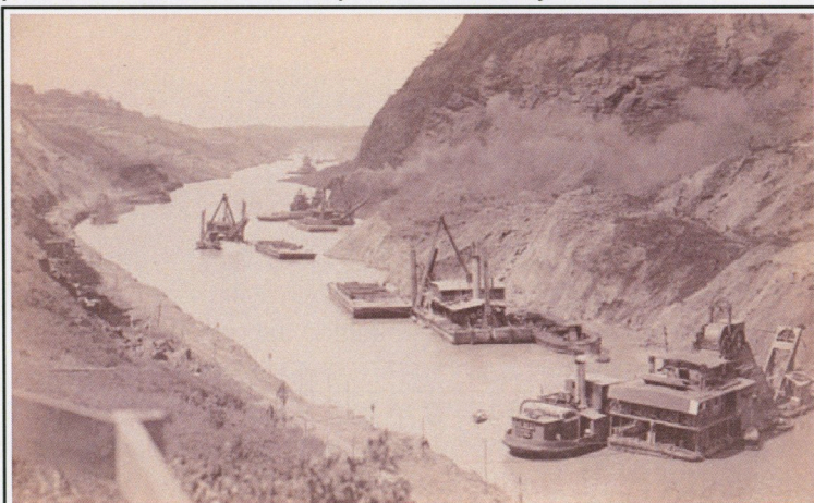
Fig. 6-4--Dredges clearing Cucaracha slide, July 1914
